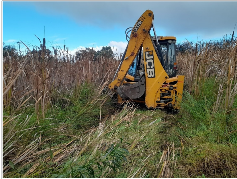
Figure 3.2: Present site conditions south-eastern portion
