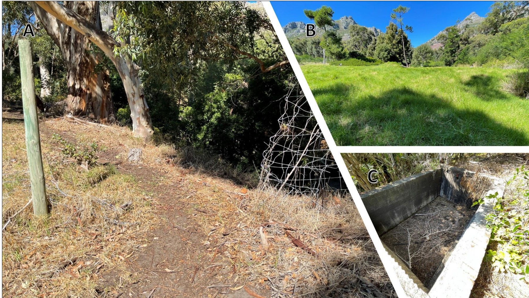
Figure 3: Some of the impacts identified in the project area: A) Footpaths and fencing; B) Severe encroachment of alien invasive plant species in wetland areas in the southern portion of the project area; and C) Old infrastructure adjacent to the Bokkemanskloof River.
