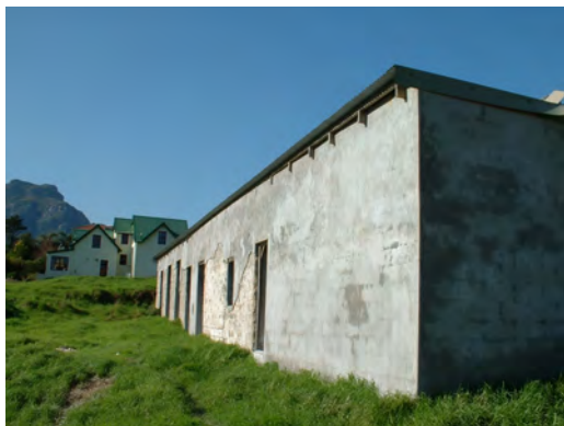
Stables in central part of the property
