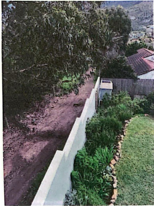
Figure 4: Photograph depicting old the proximity of the construction route and residential properties, taken in September 2024
