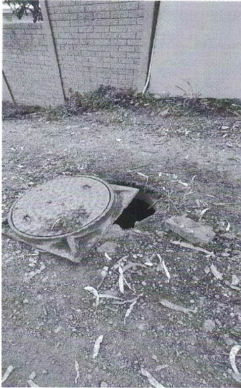
Figure 3: Photograph depicting condition of the proposed construction access route and exposed man hole, taken in September 2024
