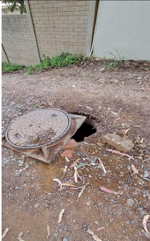
Figure 3: Photograph depicting how close this road runs to my property, no verge at all. It also shows the condition of the proposed construction access route and exposed man hole, taken in September 2024
